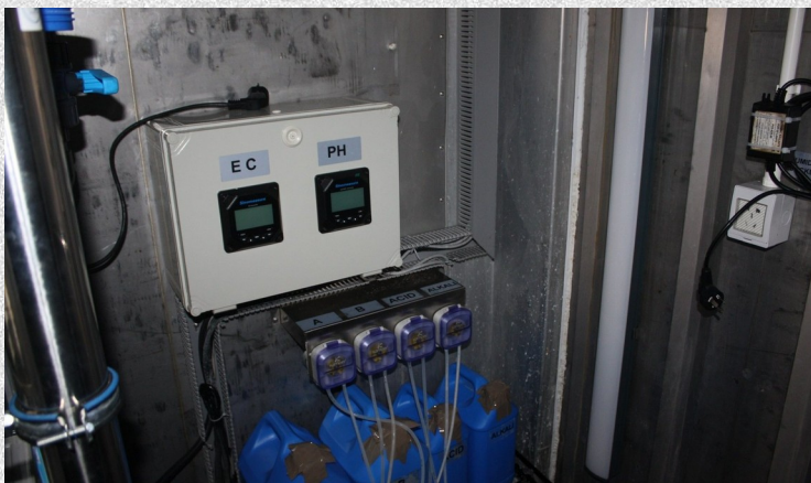
EC / PH UNIT AND PERISTALTIC DOSING PUMPS
